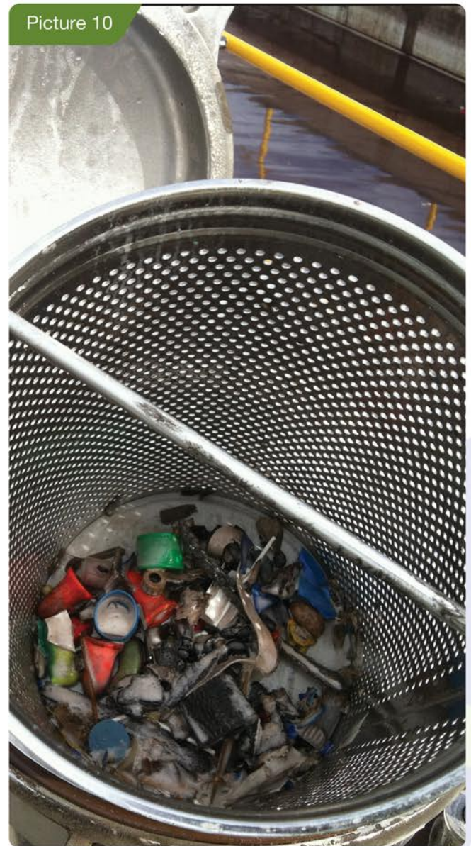
UltraSpin strainers in action removing debris.
